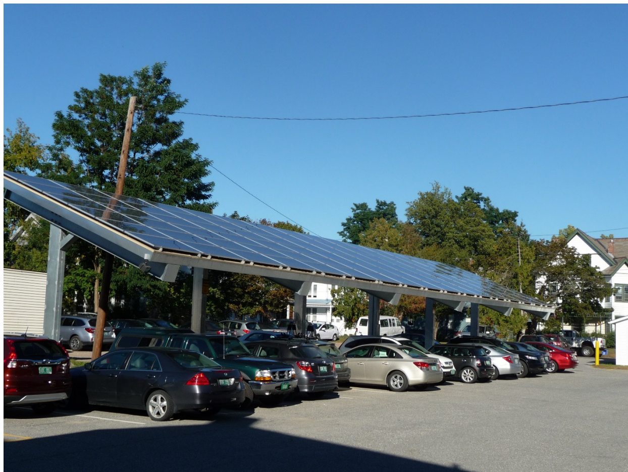
Figure 8. Solar panels installed over parking spaces at the Unitarian Universalist Society in Burlington.
